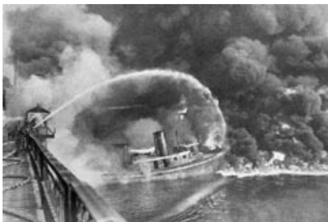
Photo courtesy of the Cleveland Public Library
